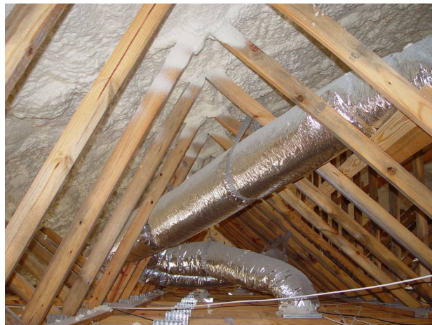
Figure 3 - Unvented attic assembly using SPF insulation (Note: rafters covered to provide layer of continuous insulation) Courtesy of Spray Polyurethane Foam Alliance
